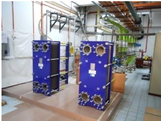
FIG. 2. New plate heat exchanger.
